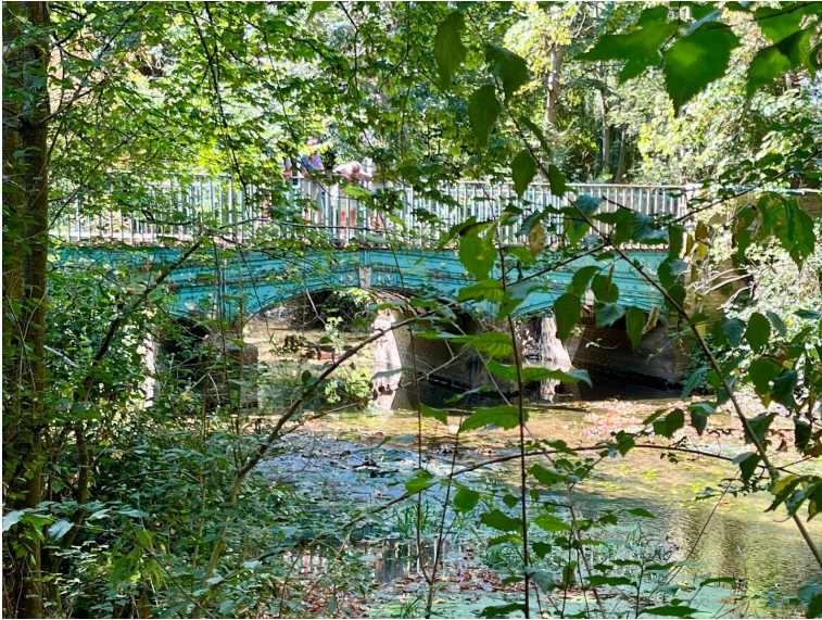
Figure 3: Bridge over River Stour
